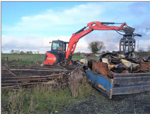
North Littleton clearance
